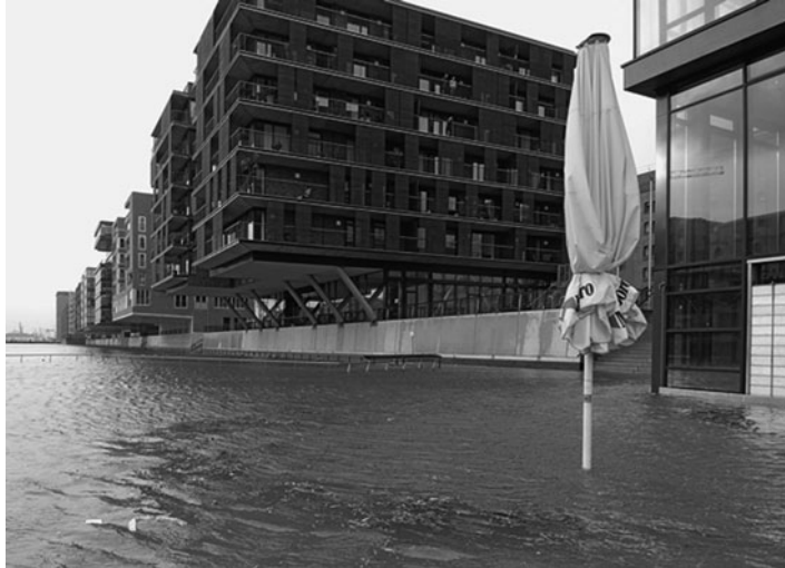
Figure 5. Basements of buildings during a storm surge in 2007. Source: ELBE&FLUT/Thomas Hampel.
